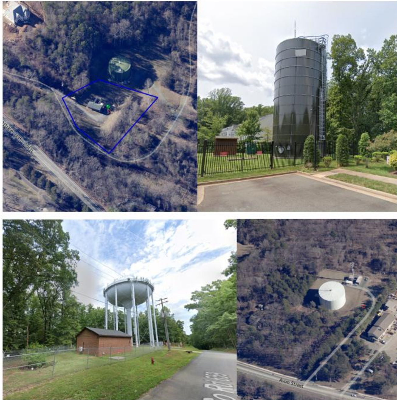
Figure 2: Water storage tanks within the County, left to right: 4466 Rockfish Gap Turnpike (Green), 1962 Tudor Ct. (Dark Green), 2226 Woodburn Rd (Light Blue), and 1737 Avon Street Ext (White).
